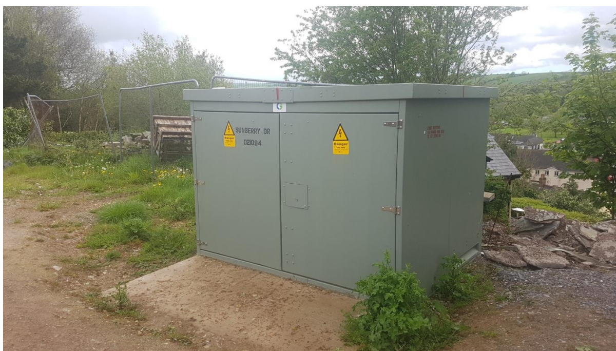
Figure 5.1 - Existing ESB Sub-Station (Sunberry Drive 02109/4)
